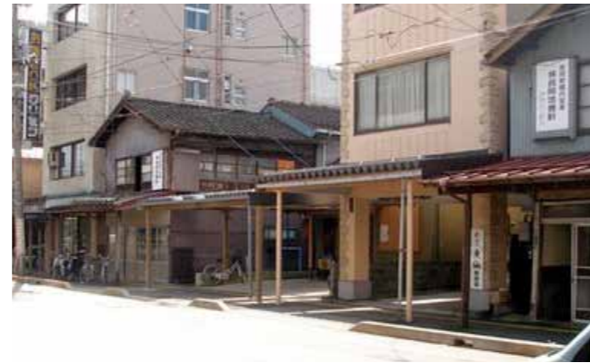
取り壊されてゆく伝統的な雁木 Gangi (covered alley), which are currently facing demolition
